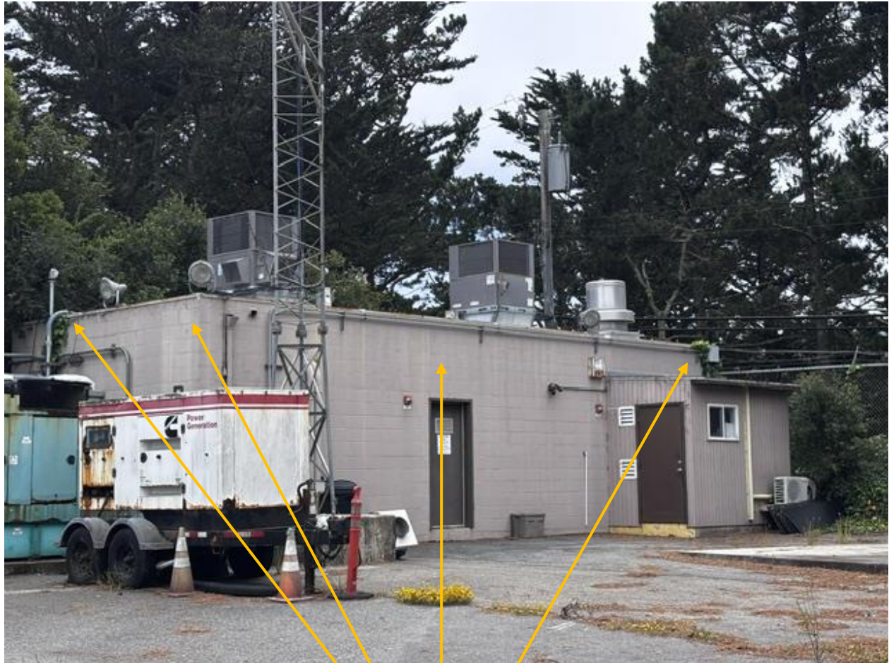
140 Arbor Ct. Radio Structure
