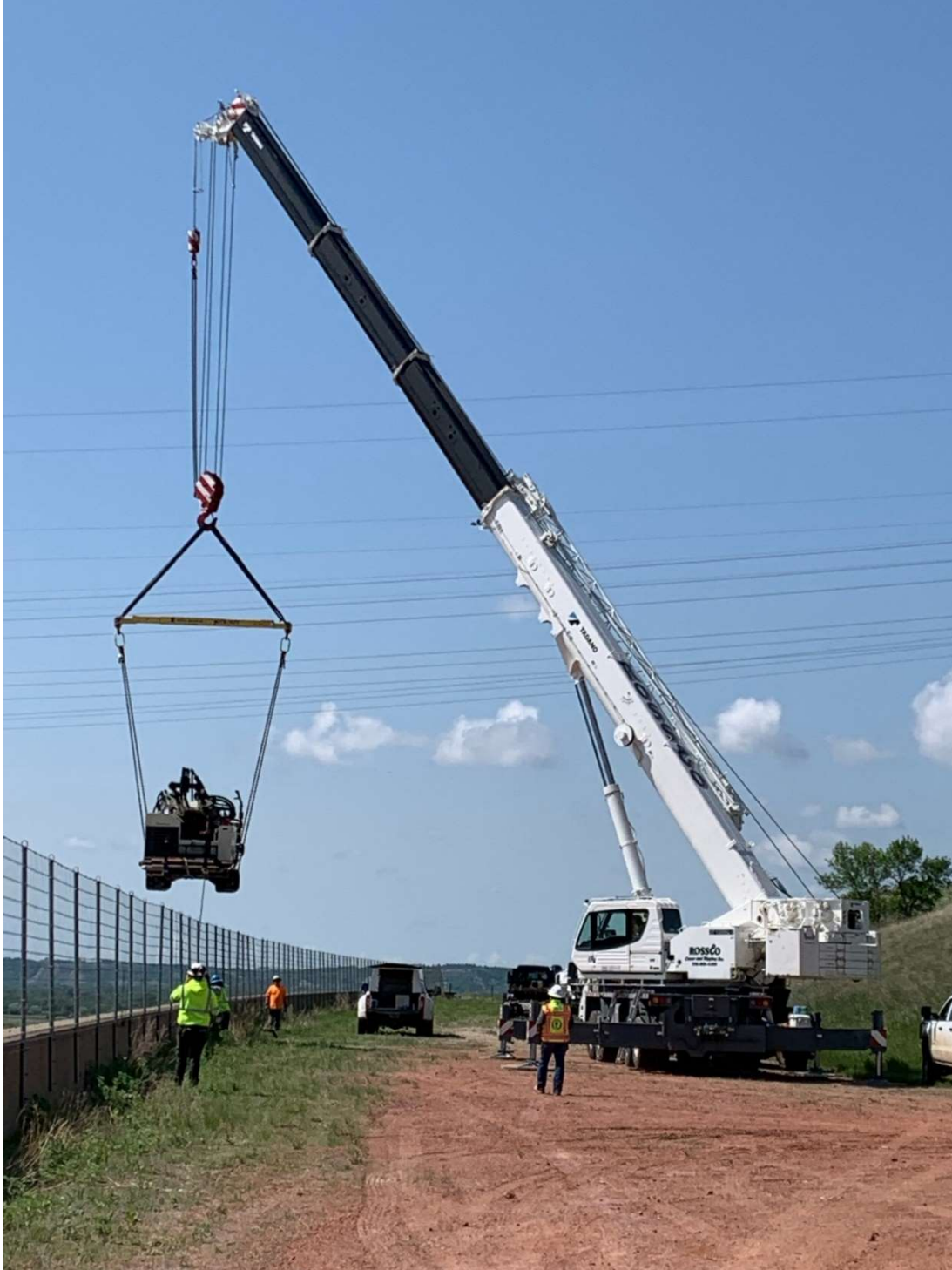
Crane placing equipment on spillway slab, circa 2025.
