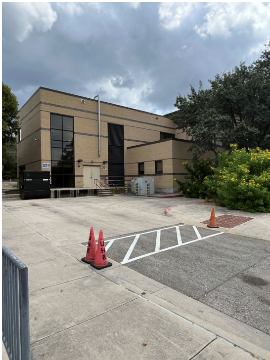
Fig. 03 Loading Area (East Side)
