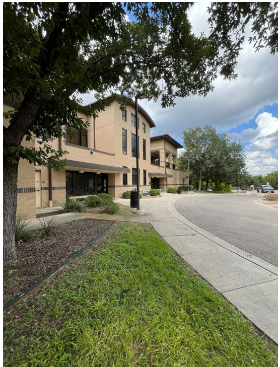
Fig. 04 Building Front (Looking East)
