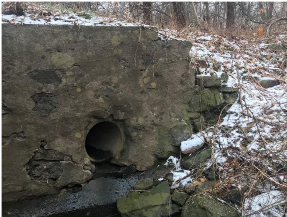
18 in. Concrete Drainage Pipe
