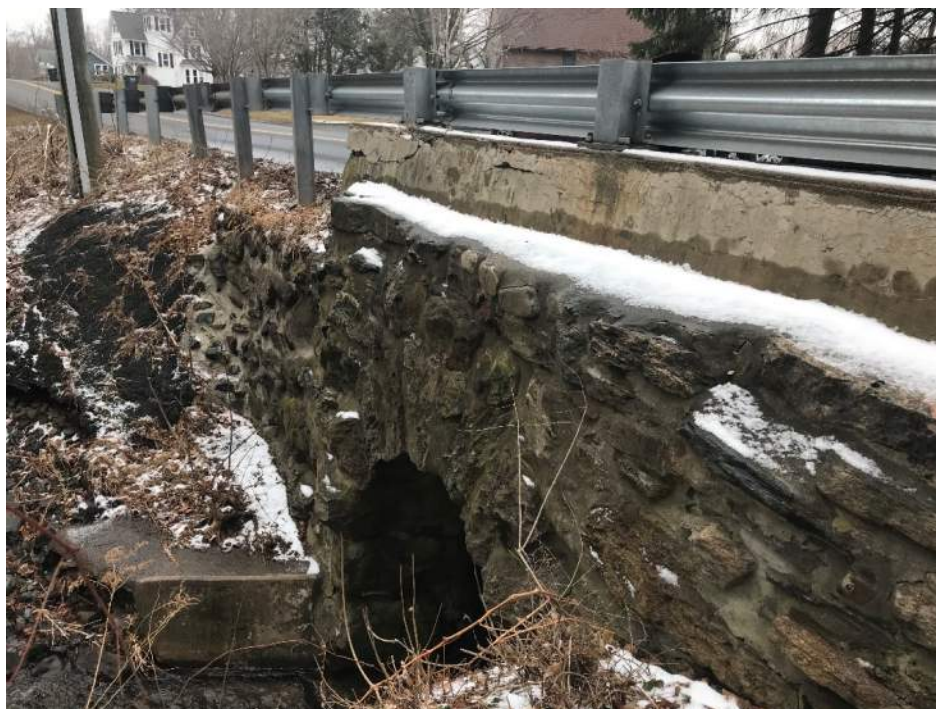
Stone Masonry Headwall at Inlet
