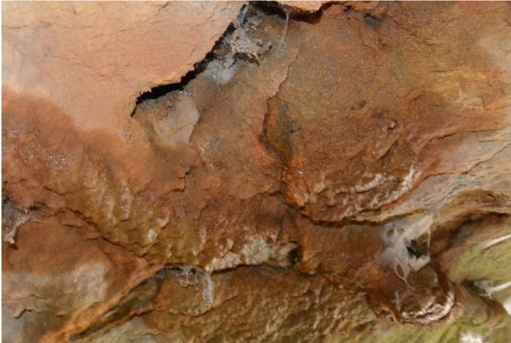
Voids in top of Stone Masonry Arch
