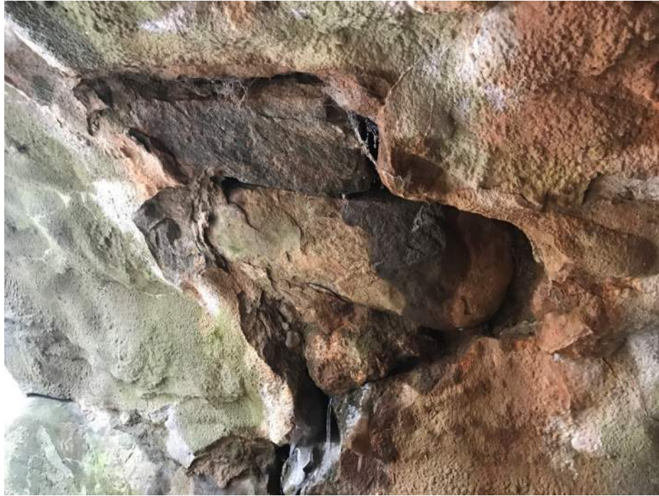
Water Damage at Stone Masonry Arch
