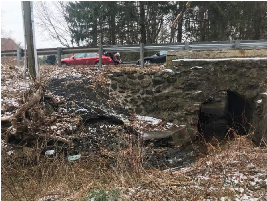
Erosion of Embankment at Inlet
