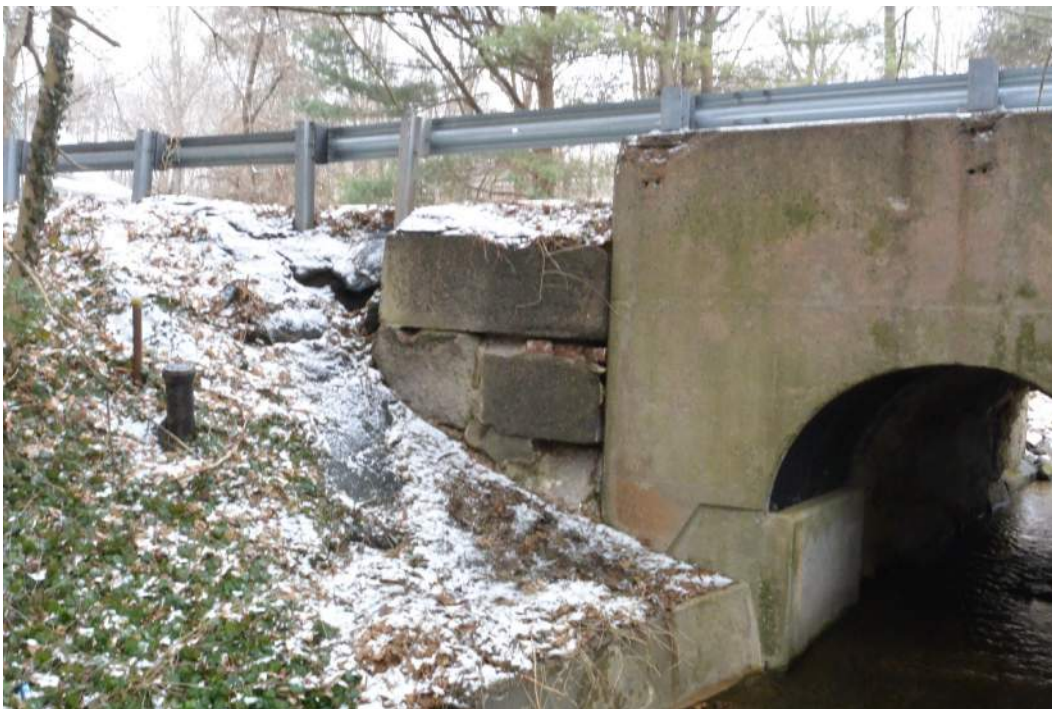
Downstream Bank - Deteriorated Precast Concrete Block Wall
