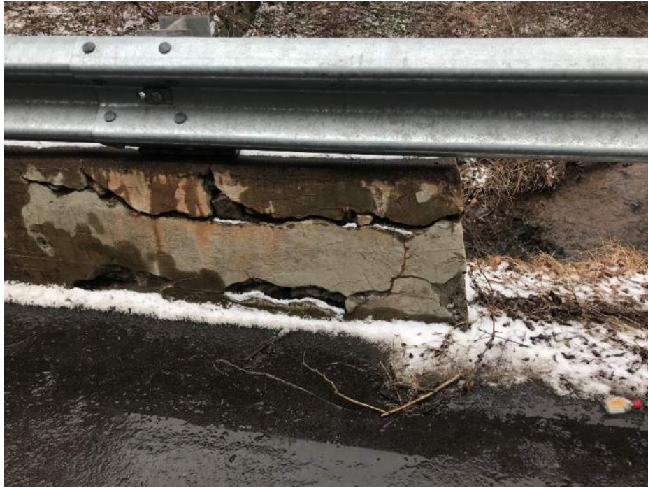
Cracked Concrete Headwall at Inlet
