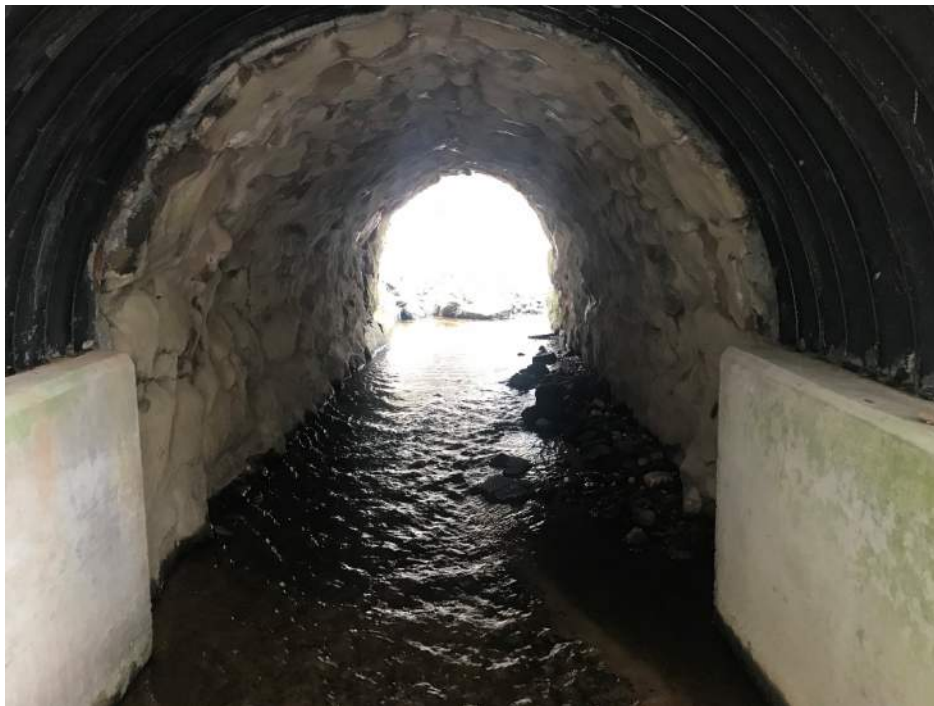
CMP Arch and Stone Masonry Arch
