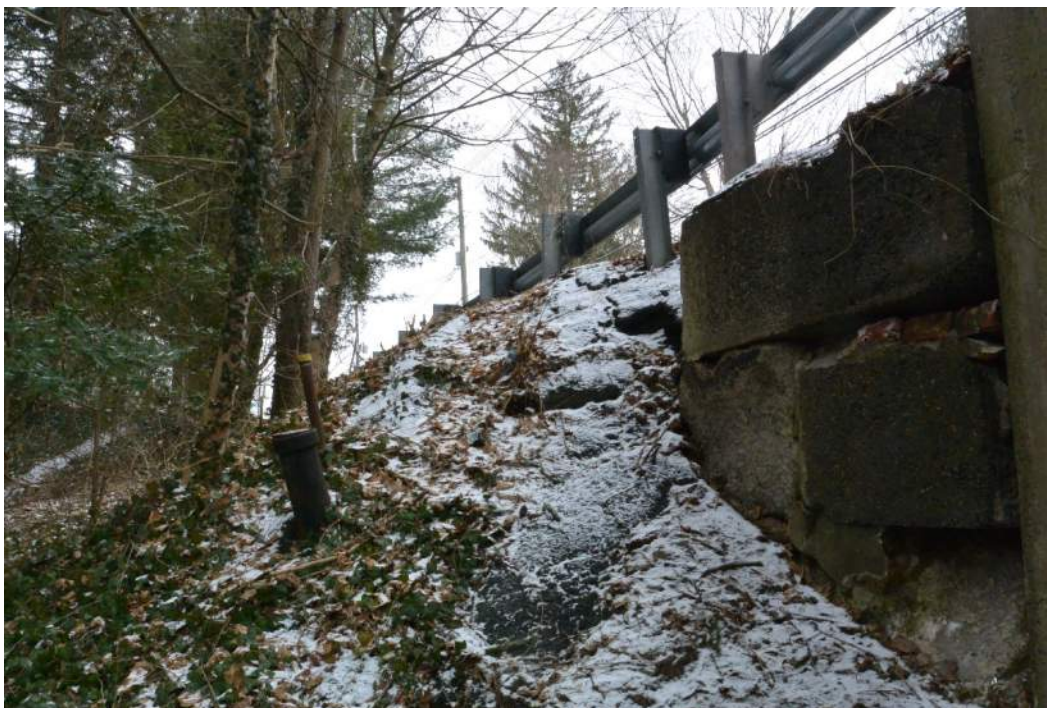
Downstream Precast Concrete Block Wingwall at Outlet
