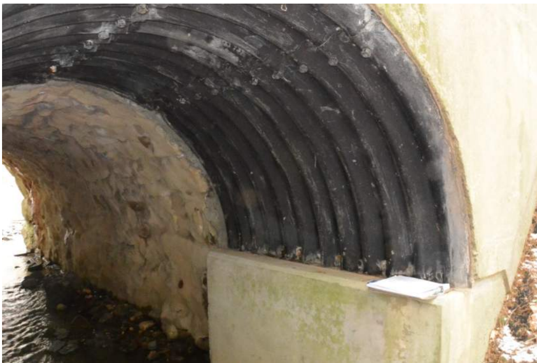
ACMP Arch on Concrete Walls at Downstream end of Structure
