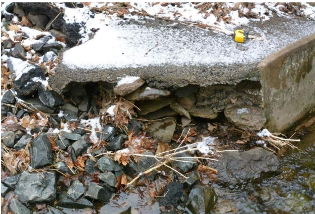
Undermined Concrete Armoring at Inlet
