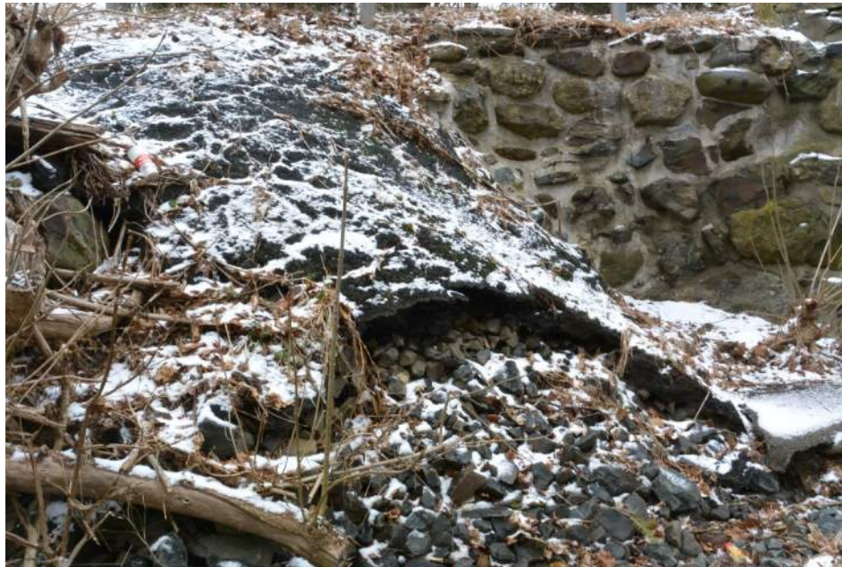
Undermined Armoring at Upstream Bank
