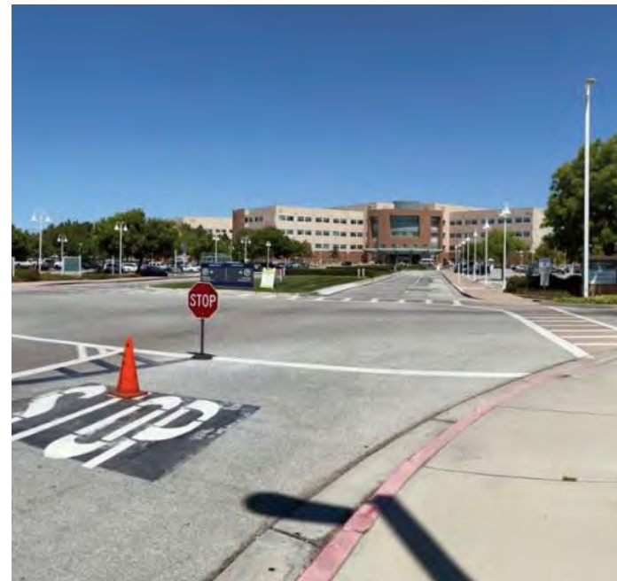
Figure 10.2.2-9. At the first intersection at PAD, directional signage is missing or not visible.
