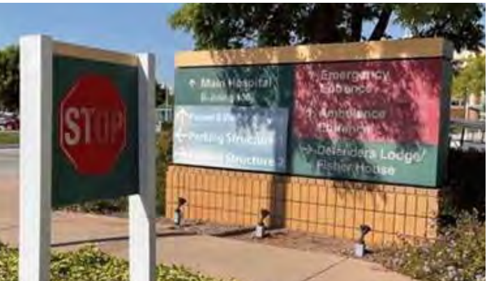
Figure 10.2.19-62. The primary directional sign at the entrance to PAD is difficult to read from a vehicle. It is faded, in shadow, and has poor contrast.
