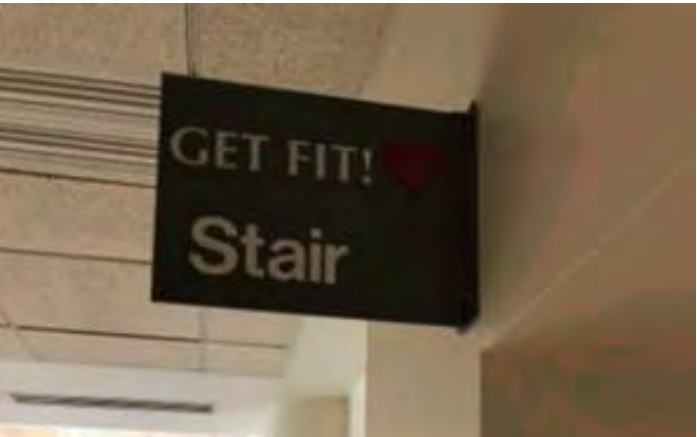
Figure 10.3.3-12. (PAD B100) The signage for these stairs labeled as “Get Fit” causes confusion: are they only for exercise or for the user to go from floor to floor? The “Get Fit” logo is not legible enough as it uses a font with thin strokes. The sign itself is lit ineffectively.
