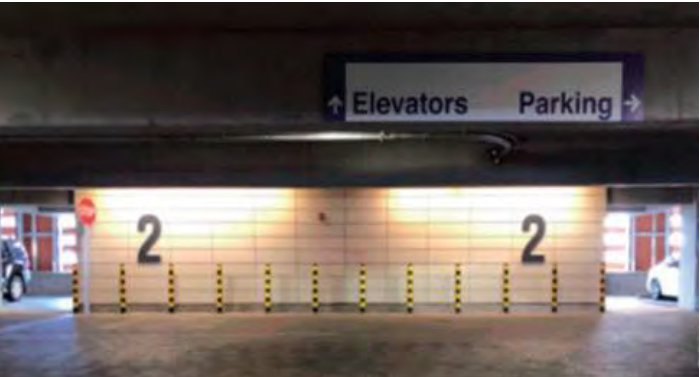
Figure 10.2.9-35. This large wall at the back of the elevator bank provides a place where wayfinding signage can go. It needs to be carefully thought out. The numeral “2” does not make it clear if it is Parking Structure 2 or Level 2. Both should be identified.
