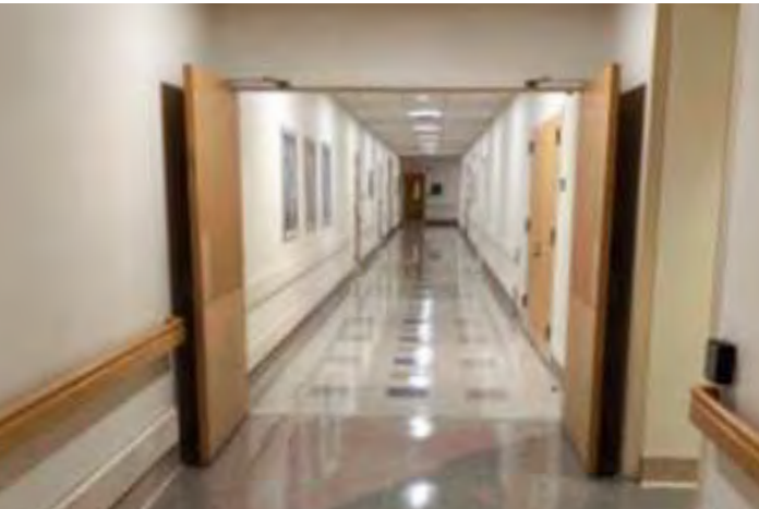
Figure 10.3.4-13. (PAD B101) There is no information about what is located down this hallway: no identification information on the soffit and no projecting signs. (Unfamiliar staff, as well as patients and families, need to know where they are going.)
