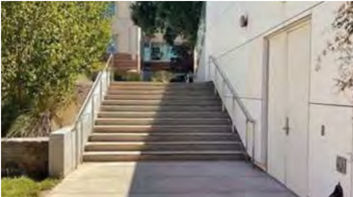
Figure 10.2.15-49. The primary route between Buildings 530 and 100/101 at PAD, includes a stairway with no signage about the location of an alternative accessible entrance.
