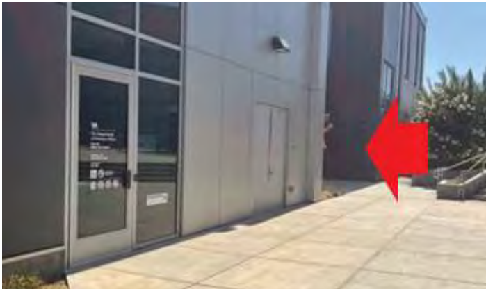
Figure 10.2.12-41. The recessed entrance to Building 105 at PAD is invisible to pedestrians and difficult to find.
