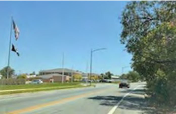
Figure 10.2.1-4. The main entrance to PAD lacks any identification signage visible to drivers approaching from Miranda Ave.
