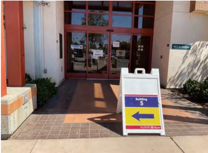
Figure 10.2.12-42. At PAD Building 7 the main entrance was closed, but the sign has nothing to do with an alternative entrance.
