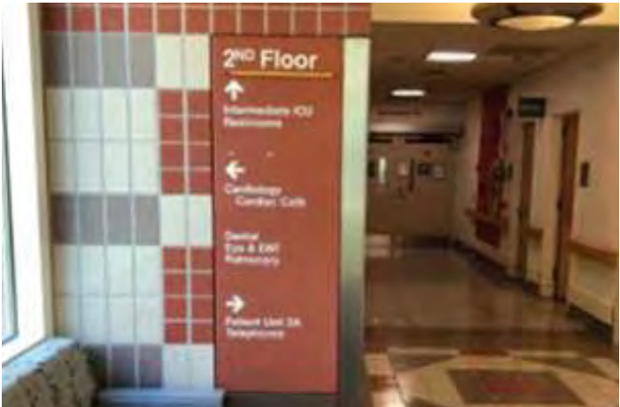
Figure 10.3.4-14. (PAD B100) The color of this directional sign on Floor 2 of Building 100 matches the color on the wall, which makes the sign less legible than it needs to be.
