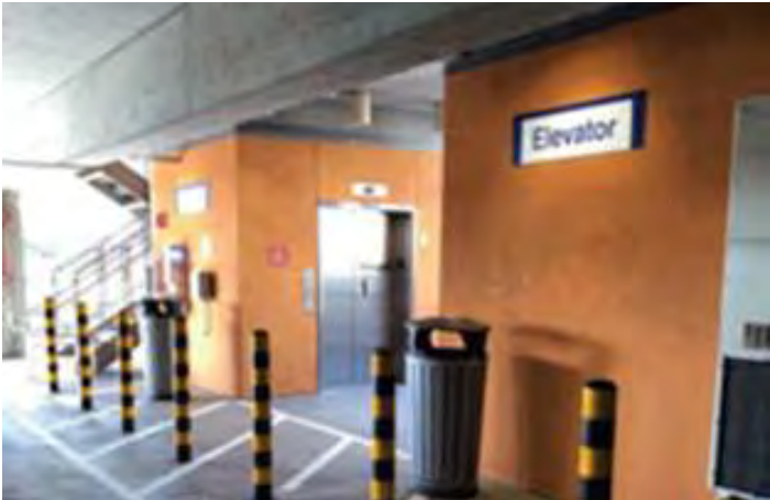
Figure 10.2.9-32. All garage levels at the elevator bank use the color orange. It may be helpful finding the elevator and stairs but unfamiliar users will misuse the color to find their cars afterwards.
