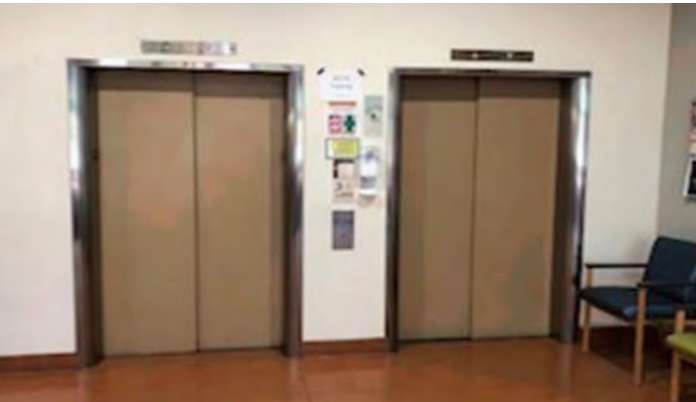
Figure 10.3.3-11. The elevators are not identified (public? Staff?) so there is no way to tell the intended users. There is no elevator directory, so it's not possible to know what floors and destinations it accesses.
