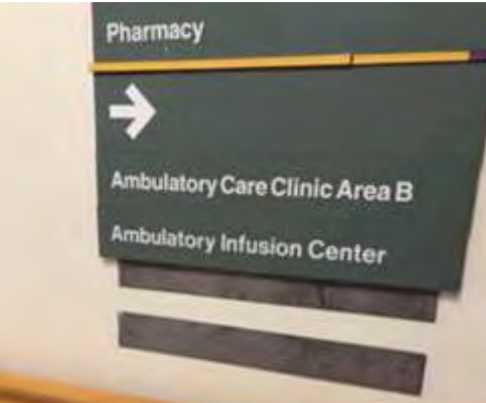
Figure 10.3.13-33. (PAD B100) A piece of the sign has fallen off or been removed and has not been replaced. This detracts from the professional look of the sign system.
