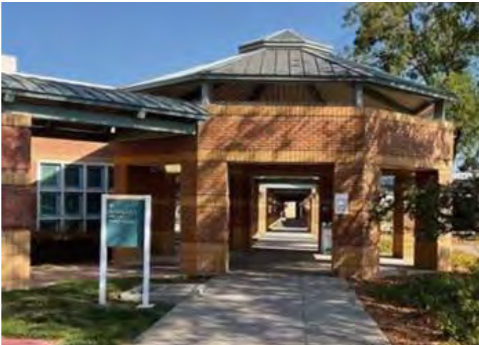
Figure 10.2.16-57. The covered walkway and intersecting “Pavilion” at PAD are a primary route between buildings but lacking a name they are seldom used for giving directions.
