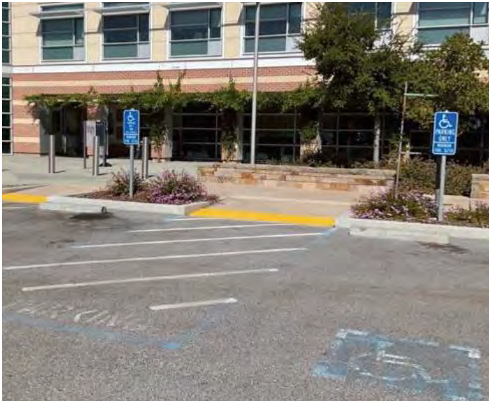
Figure 10.2.8-24. Some accessible parking spaces at PAD and MPD are missing some code required features such as visible pavement markings.
