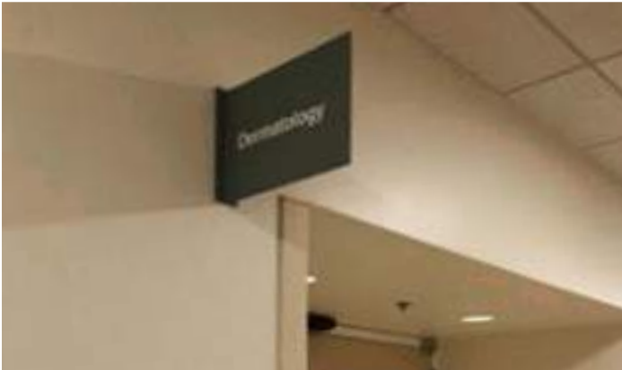
Figure 10.3.3-4. The Dermatology entrance in PAD B100 is not legible. Since this is a major department, one would expect a more formal (and legible) identification sign, like that for Radiology. This door looks like a “staff only” entrance.
