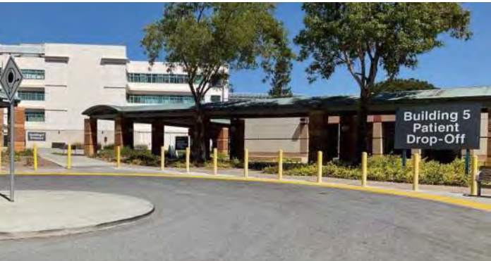
Figure 10.2.6-15. The entrance to Building 5 is not visible from the drop-off area.
