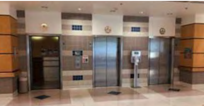
Figure 10.3.3-10. (PAD B100) These elevators are not identified by name or number. There is no indication of the intended users. There is no elevator directory, which would be useful.
