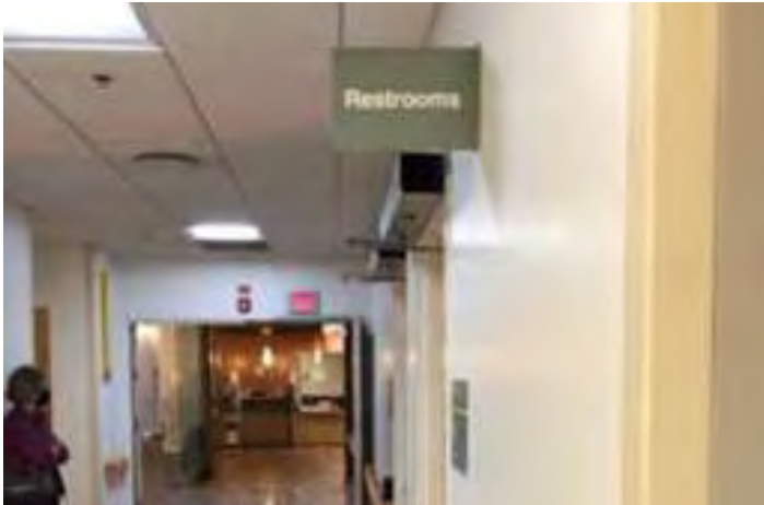
Figure 10.3.3-8. (PAD B100) The projecting ID sign for this ADA restroom does not show that it is accessible.
