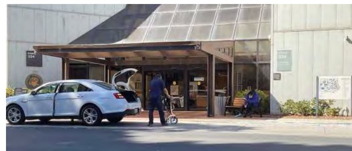
Figure 10.2.6-20. The front entrance of MPD Building 334 is not well identified. It needs a larger identification sign and directional.
