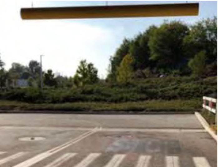
Figure 10.2.9-37. There are no directional signs on the Loop Road at the garage exits.
