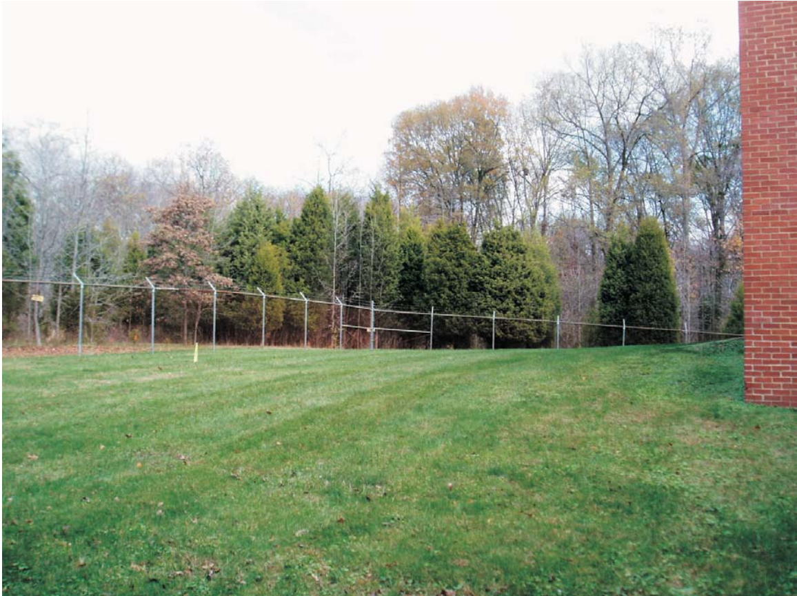
Figure 15. The portion of the temporary easement area that is within the pumping station yard, facing northwest.
